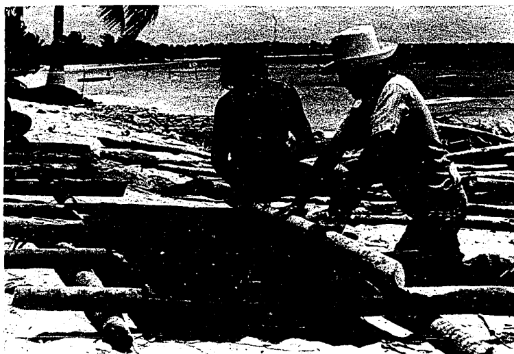
Fig. 5.20. Construction of a casita de tambo , with a flattened barrel side for "roof."
