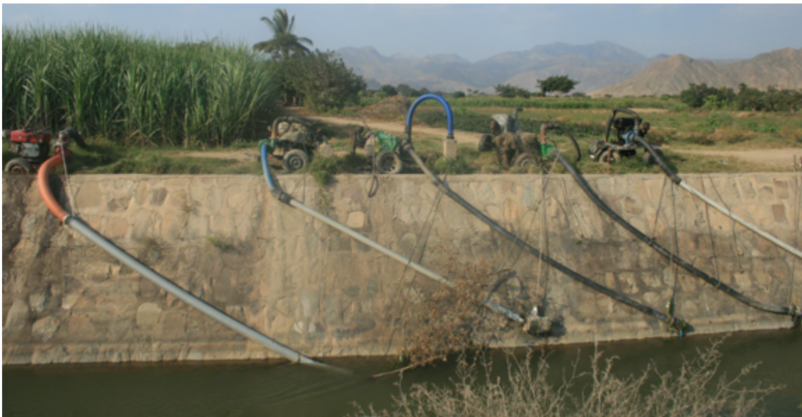
Figure 2. Headenders' Pumps in the Taymi Canal
