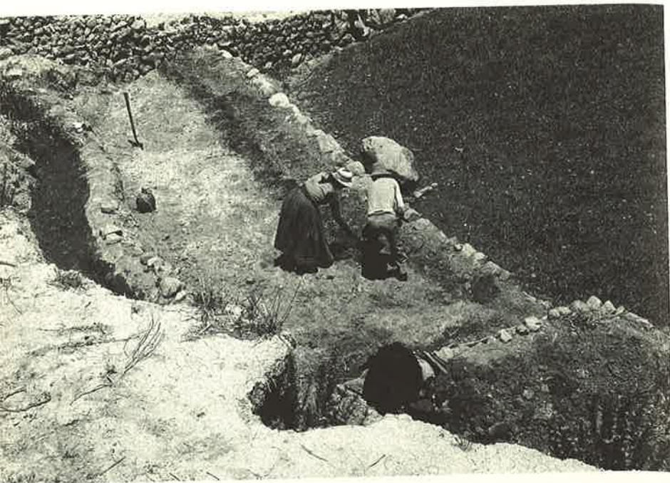
Rebuilding terraces and canals
